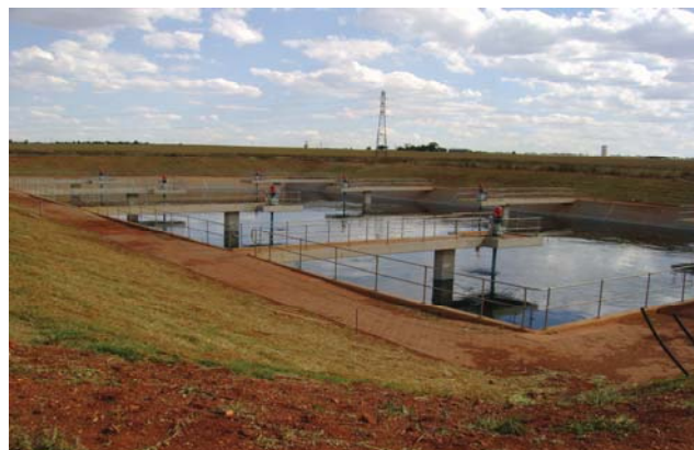
The new off-line balancing dam at Hartebeestfontein WCW
