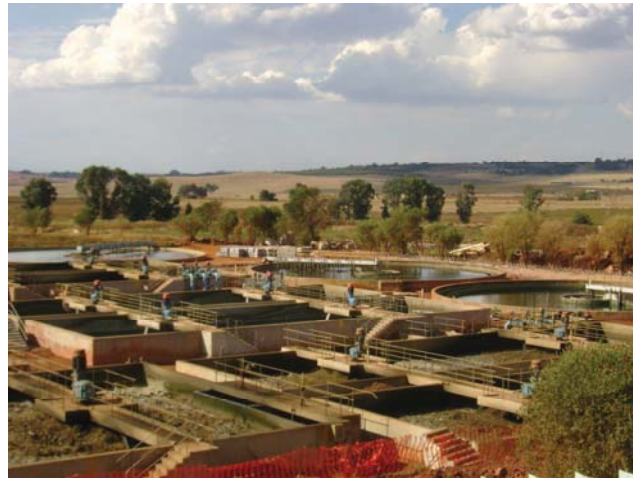
Hartebeestfontein WCW being upgraded
